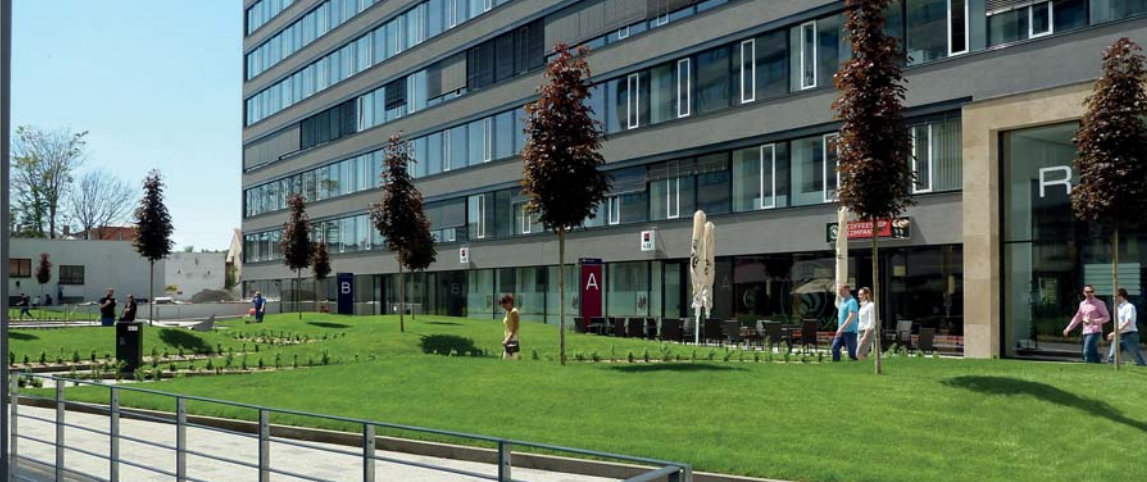
Titanium Brno - realizace GreenVille service Brno
